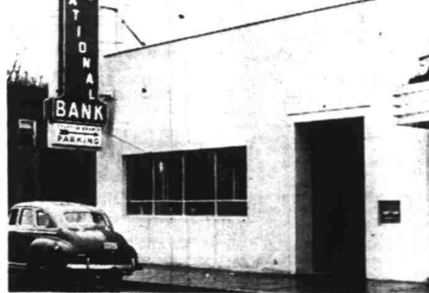
STAYTON—Stayton's branch of the First National Bank of Portland is celebrating its 15th birthday by opening for business in a new building on Third street in the downtown district. The photos show the exterior and the flower-decked interior. (Statesman photos).
