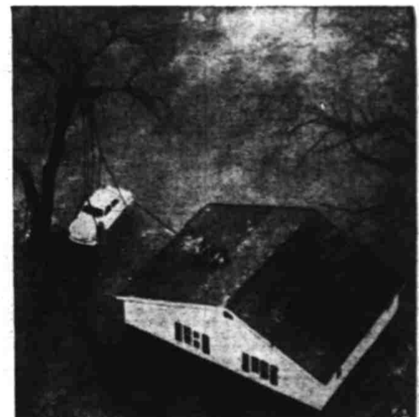
AFTER THE DELUGE —In 1950's major flood last May in Winnipeg, Manitoba, necessity was the mother of invention as this car owner rigged up a rope and pulley from a tree to save his car, while bicycles were lashed to the roof of his home.
