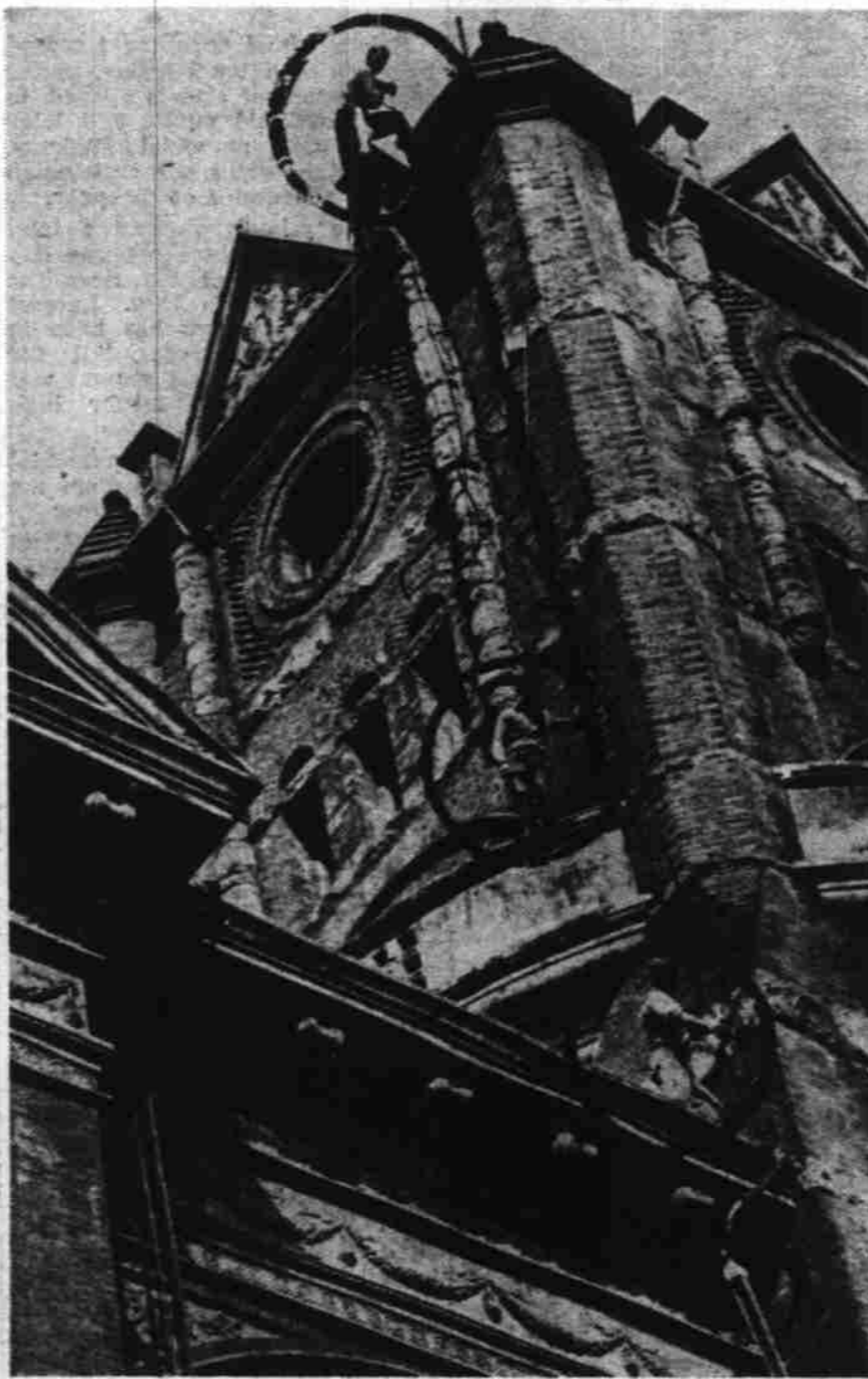
Three men on a tower—as circled above—kept passersby craning their necks to watch the steam cleaning of Salem's city hall Monday. The Portland cleaning crew started the $5,000 wash and paint task on the east face of city hall and by afternoon had started working around the tower. Some 55 years of smoke and grime are being removed from the building, revealing the warm red color of the bricks, and lightening the gray stone work. The cleaning will take several days. (Statesman photo.)
