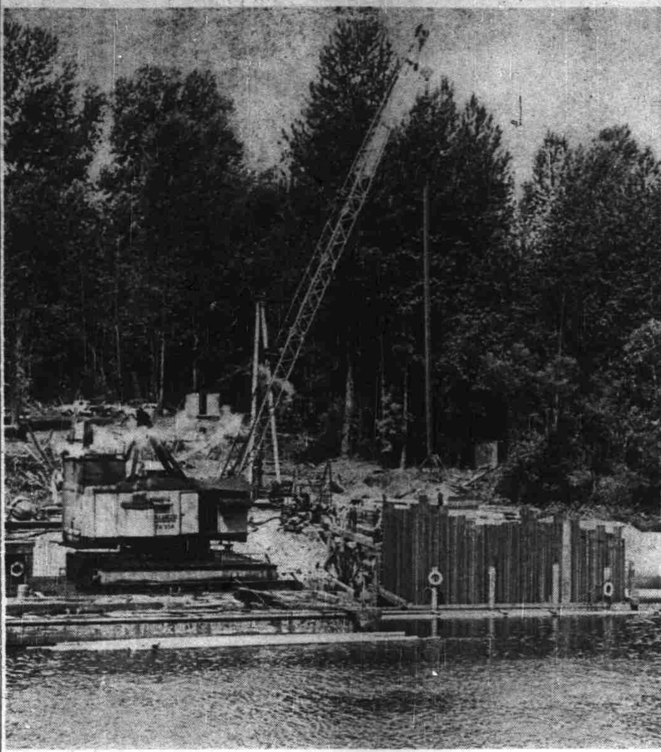
Sheet steel piling 50 feet long is being driven into the Willamette river bed to form pier cofferdams for Salem's new bridge. Here a giant crane lifts one of the piling into position where pier number four will be located. It is being driven into place as form for the pier. Excavation for pier number five is about completed and the cofferdam in place, located directly behind the pier site shown. Pier erection work is being done by Lee Hoffman, contractor. (Photo by Don Dill, Statesman photographer.)
