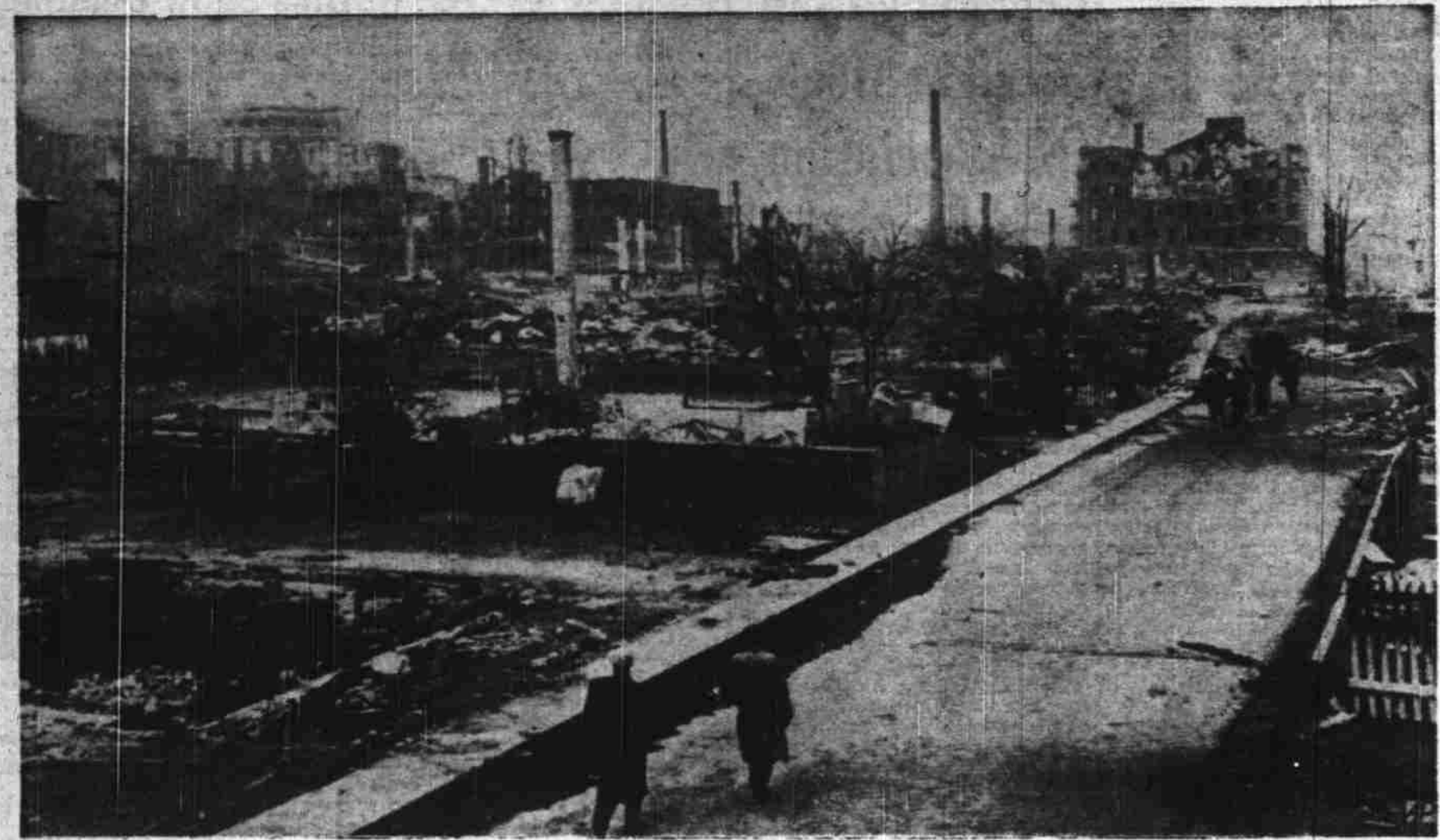
RIMOUSKI, Que., May 8—Relief workers faced the gigantic task of caring for 2,500 persons made homeless in a blaze which gutted one half of this town of 15,000 population on the St. Lawrence river. Ruins near the center of the town are pictured above. Property loss in the Sunday blaze was estimated at $20,000,000. (AP Wirephoto to The Statesman).
