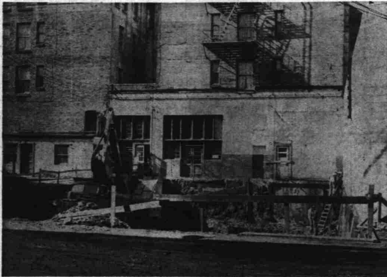
Excavation for the basement part of the Senator hotel's new addition is well under way this week. The new addition will give greater room capacity to the hotel, making one of the largest in Salem. It will occupy the space formerly used as a bus loading and unloading zone when the bus station was in the hotel. Above is a view of the area showing how the old canopy covering the loading zone has been removed at a truck being loaded by a power shovel at left. (Statesman photo.)
