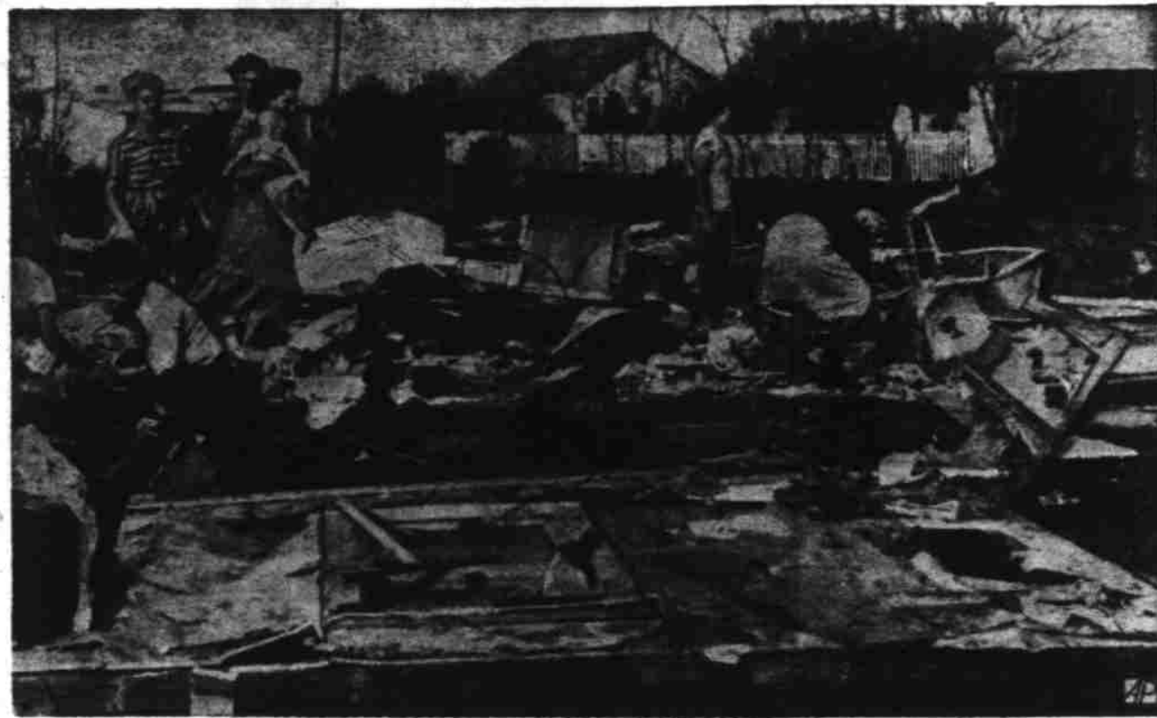
LA PORTE, Tex., Feb. 12—The home of Mr. and Mrs. H. A. Weatherford at La Porte, Texas, was completely demolished when a twister struck it. The Weatherfords received serious injuries. Relatives and neighbors are collecting scattered valuables. One person died and at least 12 were reported injured in the tornado. Twenty-five homes are listed as destroyed and about 200 homeless. (AP Wirephoto to The Statesman).
