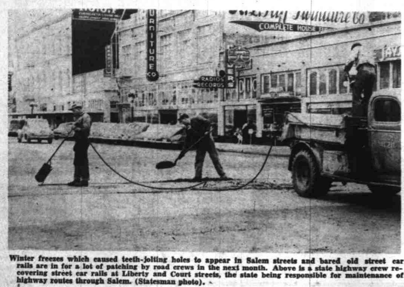
Winter freezes which caused teeth-jolting holes to appear in Salem streets and bared old street car rails are in a lot of patching by road crews in the next month. Above is state highway crew recovering street car rails at Liberty and Court streets, the state being responsible for maintenance of highway routes through Salem. (Statesman photo.)
