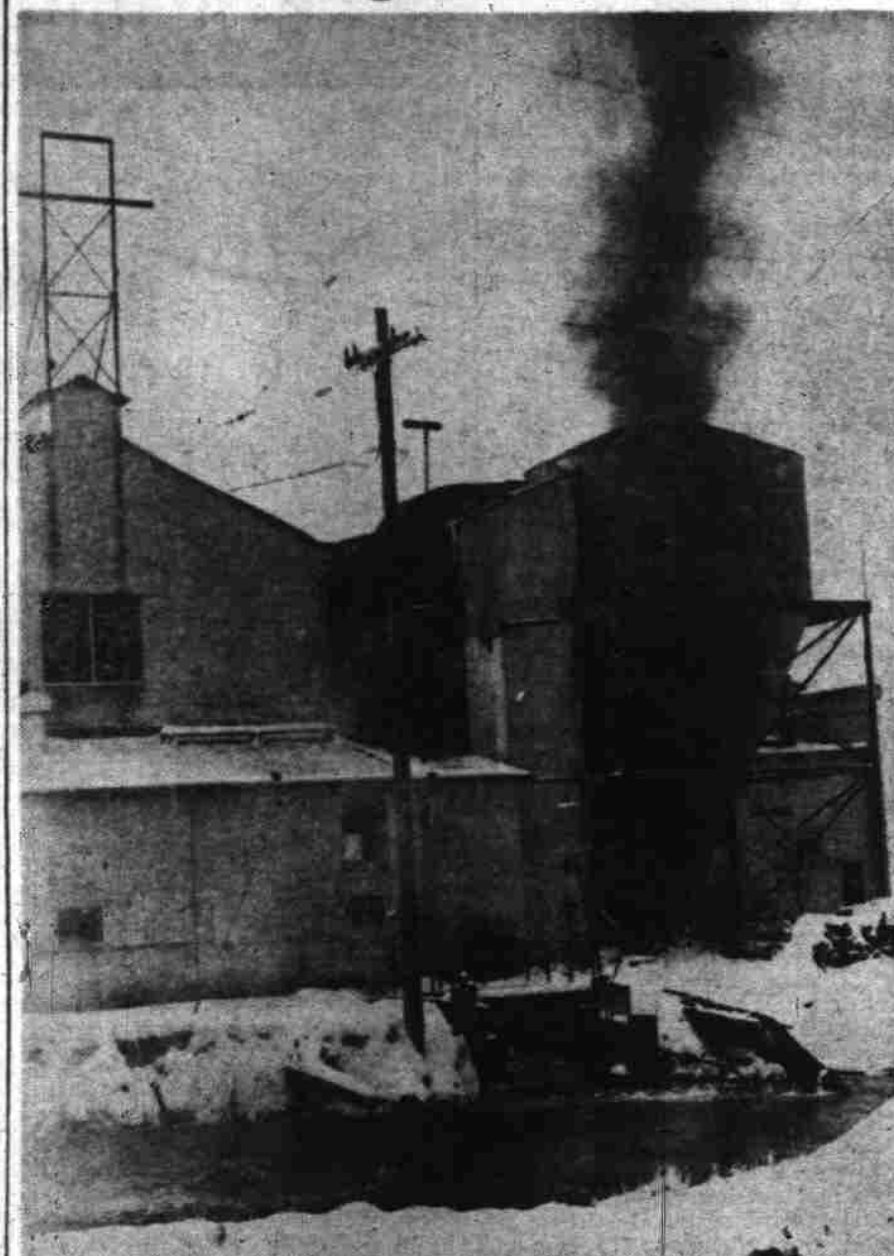
Portland General Electric's seldom-used steam generator plant at Mill and Liberty streets is being put to work these days during the extreme cold as electricity users, both domestic and commercial, take more and more electrical energy to combat the cold. Above, a cloud of black smoke comes from the boiler stack Tuesday morning when it was really cold. (Statesman photo.)
