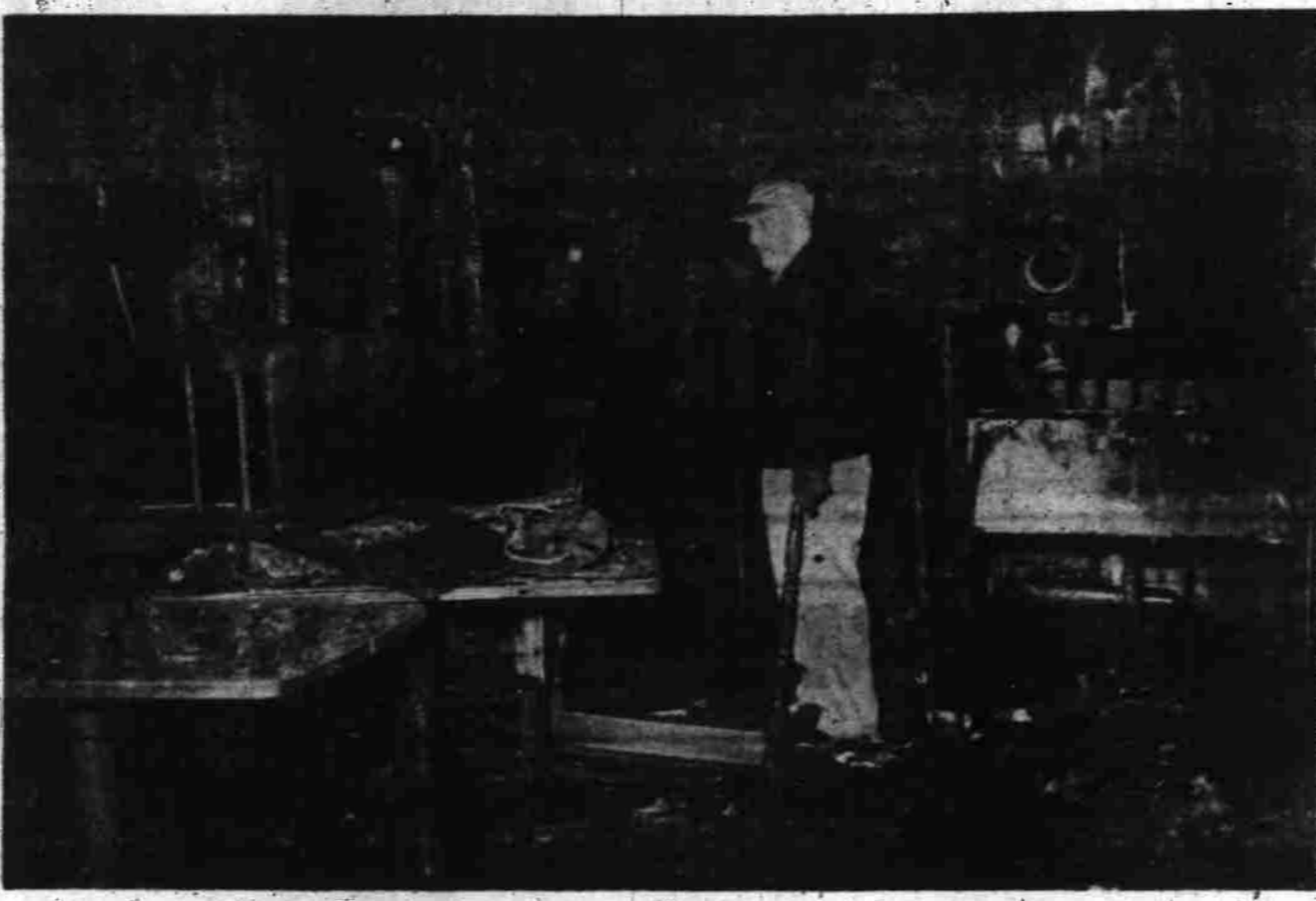
Fire left The Ranch, popular eating place at 3260 Portland road, a blackened shambles early Tuesday morning. Sub-zero temperatures hampered firemen fighting the blaze which started at 3 a. m. Above is an interior view with co-owner D. H. Williams standing near an oil circulator where fire is believed to have started. Williams' partner is D. H. Eyerley. Damage was said to be nearly 50 per cent complete, according to firemen. (Statesman photos). (Story on page 1).
