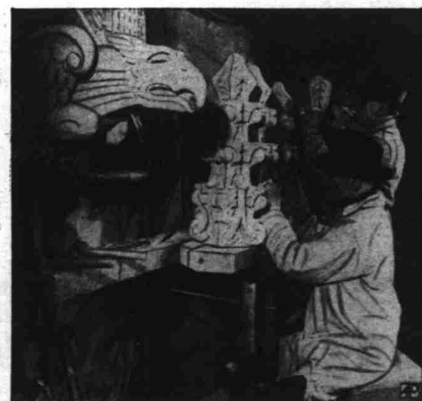
CARVING FAMILY—Kenneth Gardner (foreground) and his father, William, carve sandstone decorations for the rebuilt bomb-damaged British House of Commons in London, as work nears completion.
