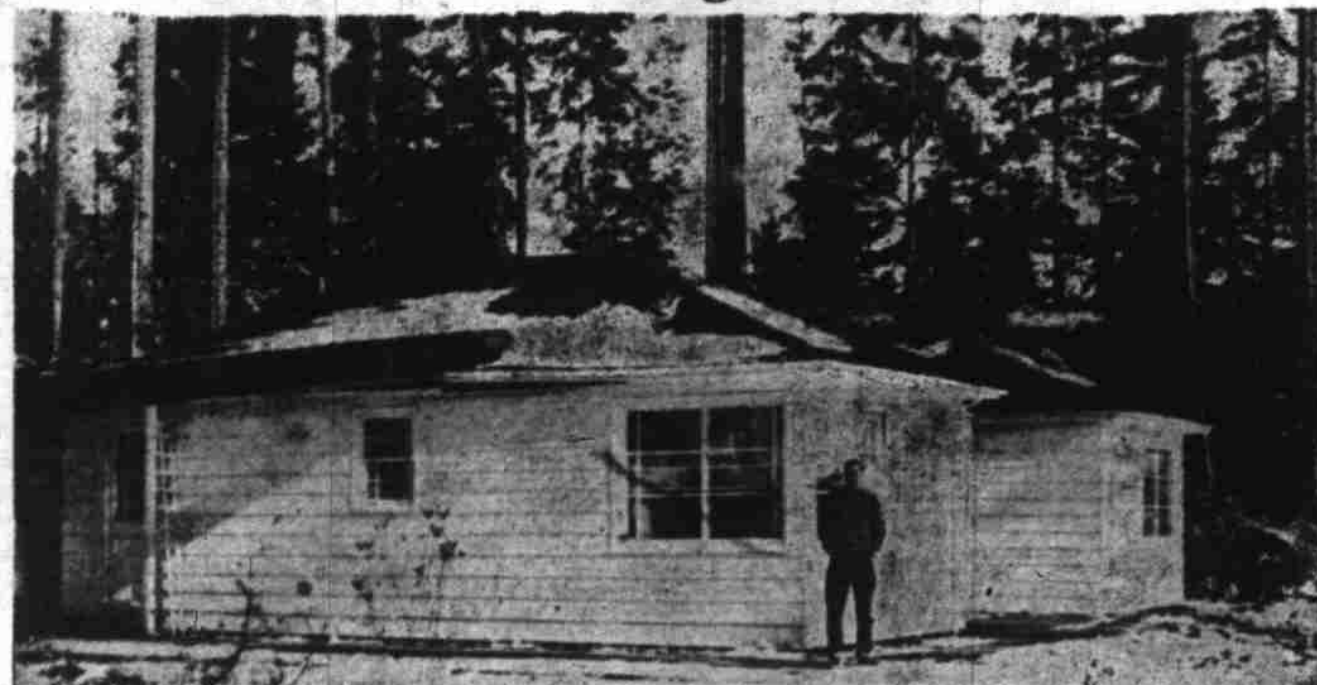
Sid Simning, 850 Bever dr., surveys the damage done to his new house just off North River road when a tall tree came crashing down on its roof. The big Douglas fir, and another one in Simning's backyard, were blown over at the height of a raging snow storm late Friday afternoon. None of the house's occupants was injured but the 20-inch, 150-foot-tall tree jarred loose several sections of the interior ceiling and ripped a hole in the front porch ceiling. A falling tree smashed Simning's car in a similar accident last winter, he said. (Statesman photo.)
