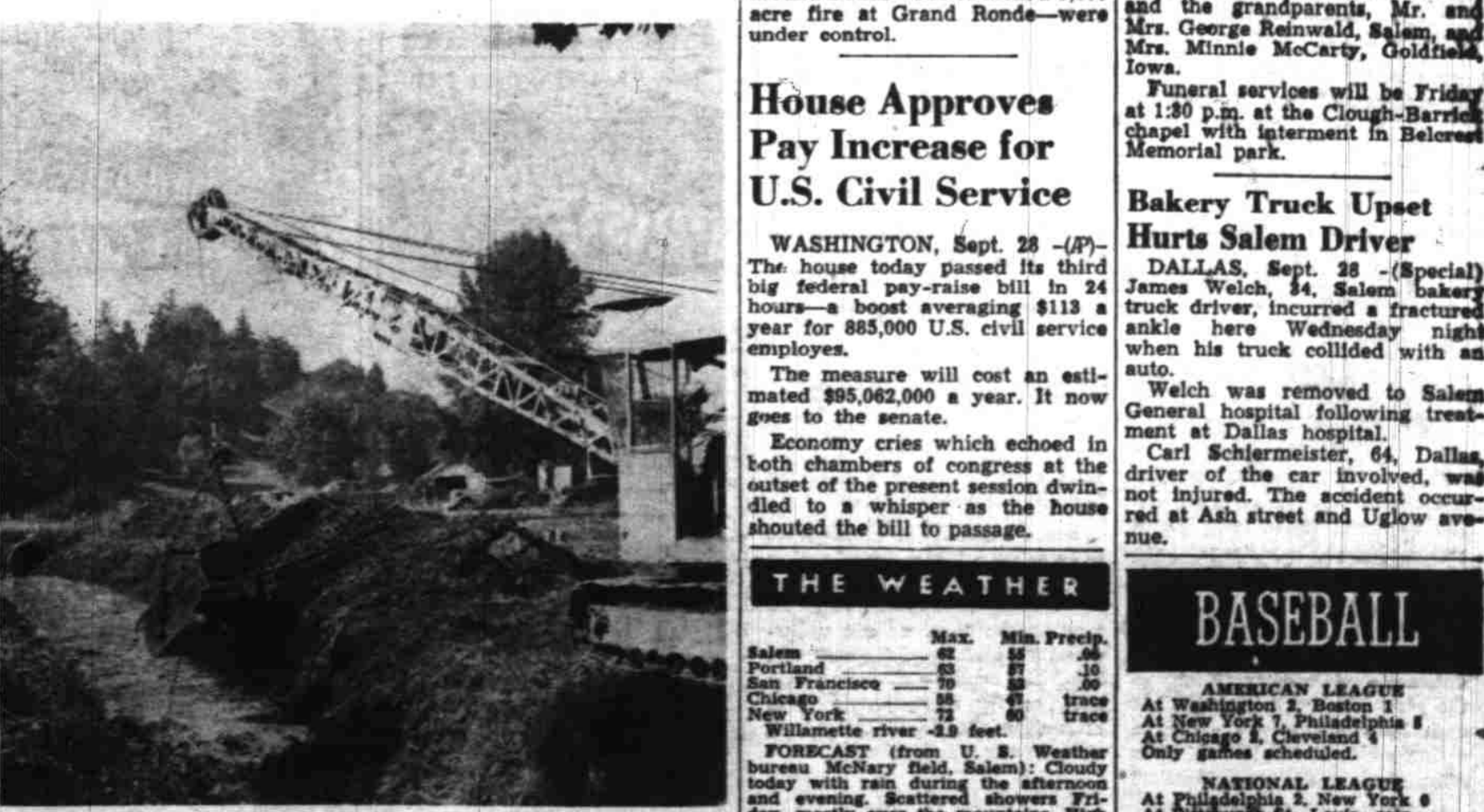
Winter rains and spring floods won't be plaguing the southeastern part of Salem this year as much as in past years if drainage work now under way is of any avail. Clearance and dredging of a channel on a ditch running in a northwesterly direction from a point about four blocks south of city limits at south 12th street past Leslie
