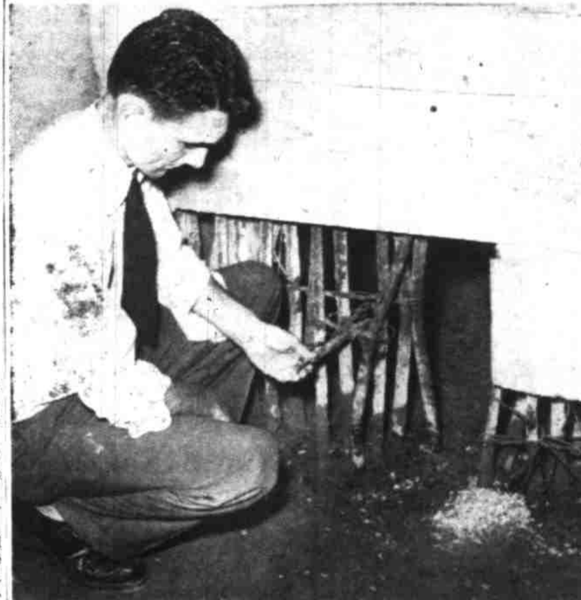
H. C. Cupp, 840 Shipping st., prison guard, inspects the small hole made in bars at wall junction of the prison wall where three convicts made their break to freedom Thursday evening. Convicts used tools taken from a locker to splinter a heavy three by twelve inch plank covering the bars, and then using concrete reinforcing wire they bent the bars by twisting the wire with a short piece of iron rod.
