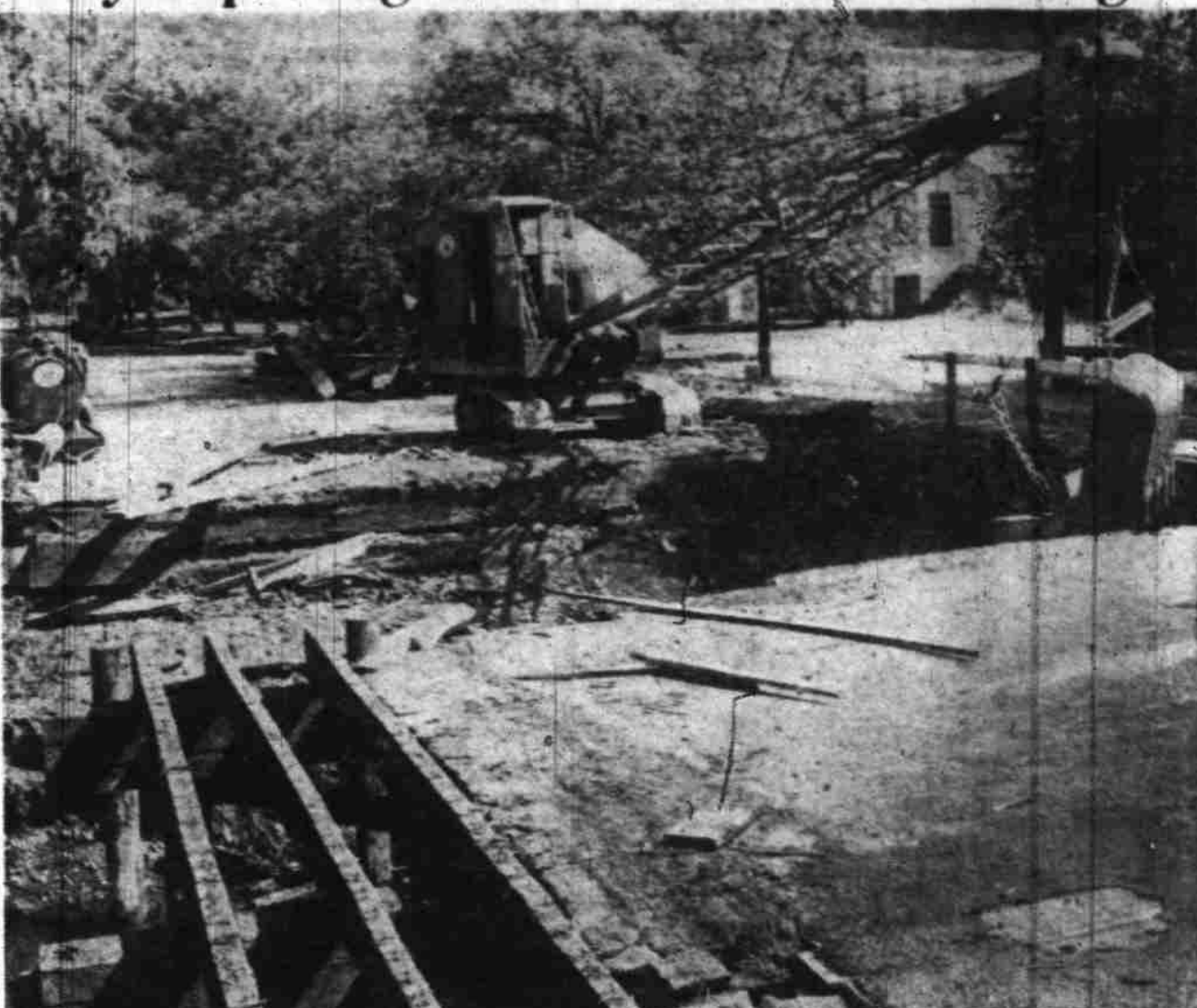
Crews are busy wrecking the old, dilapidated Mill creek bridge on North Church street between Union and D streets. Condition of the bridge was found to be badly deteriorated, as can be seen in the right foreground where rotted ends of planks showed through the pavement. A modern bridge with concrete footings will be constructed as soon as the old bridge is dismantled. (Statesman photo.)
