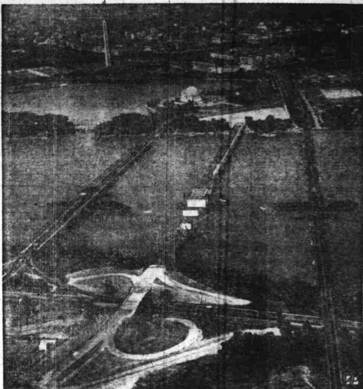
WASHINGTON BRIDGES—The new Washington 14th Street bridge is seen from the Virginia side between older bridges. Cloverleaf at bottom will channel traffic to Mt. Vernon Highway.
