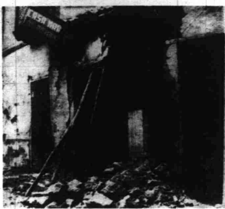
AMBATO, Ecuador, Aug. 11—Wooden poles are used to prop up the sagging wall of this store building in Ambato after it was damaged August 5 in an earthquake which claimed an estimated 6,000 lives.
