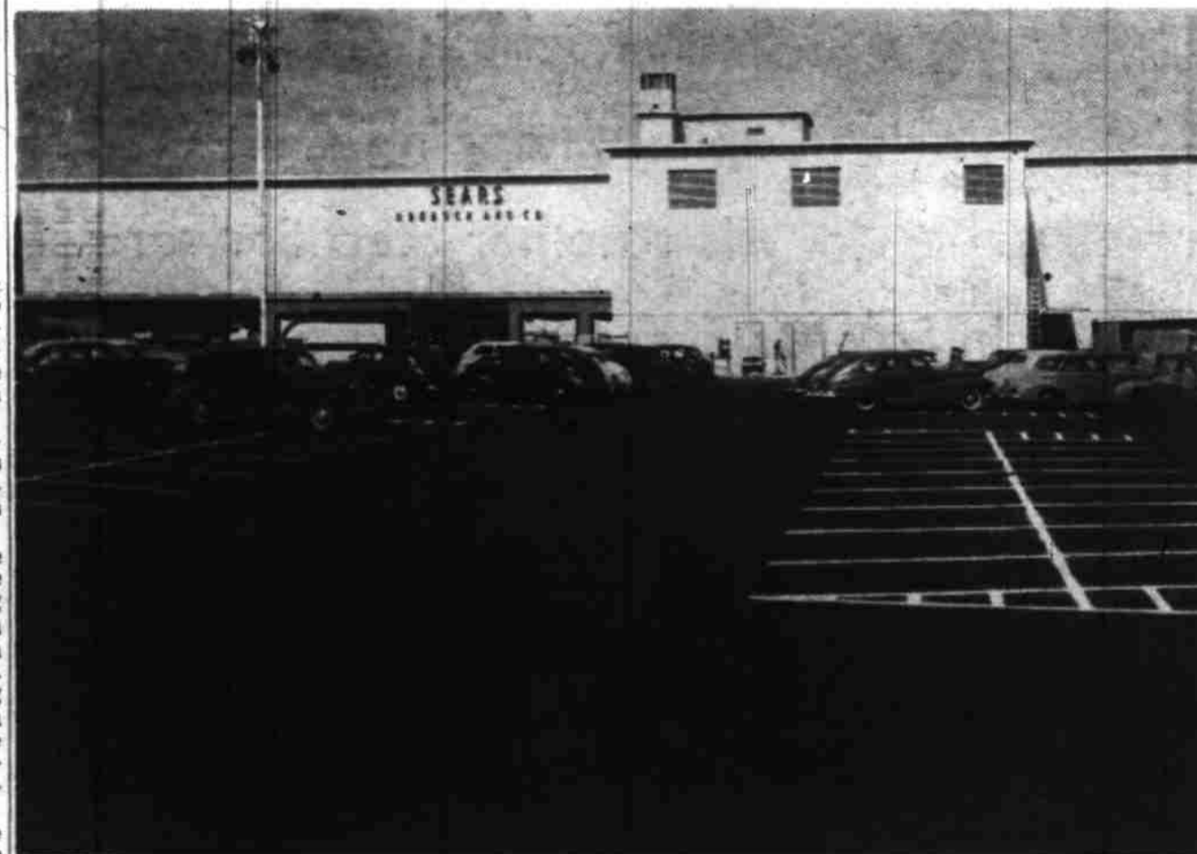
Biggest concentration of automobile parking area for some 500 cars in the new Capitol Shopping center is the 500-car parking lot partially pictured above. Located in the rear of the new Sears store which opens today, the lot is approached from Marion street, has easy-angle parking and convenient access routes.
