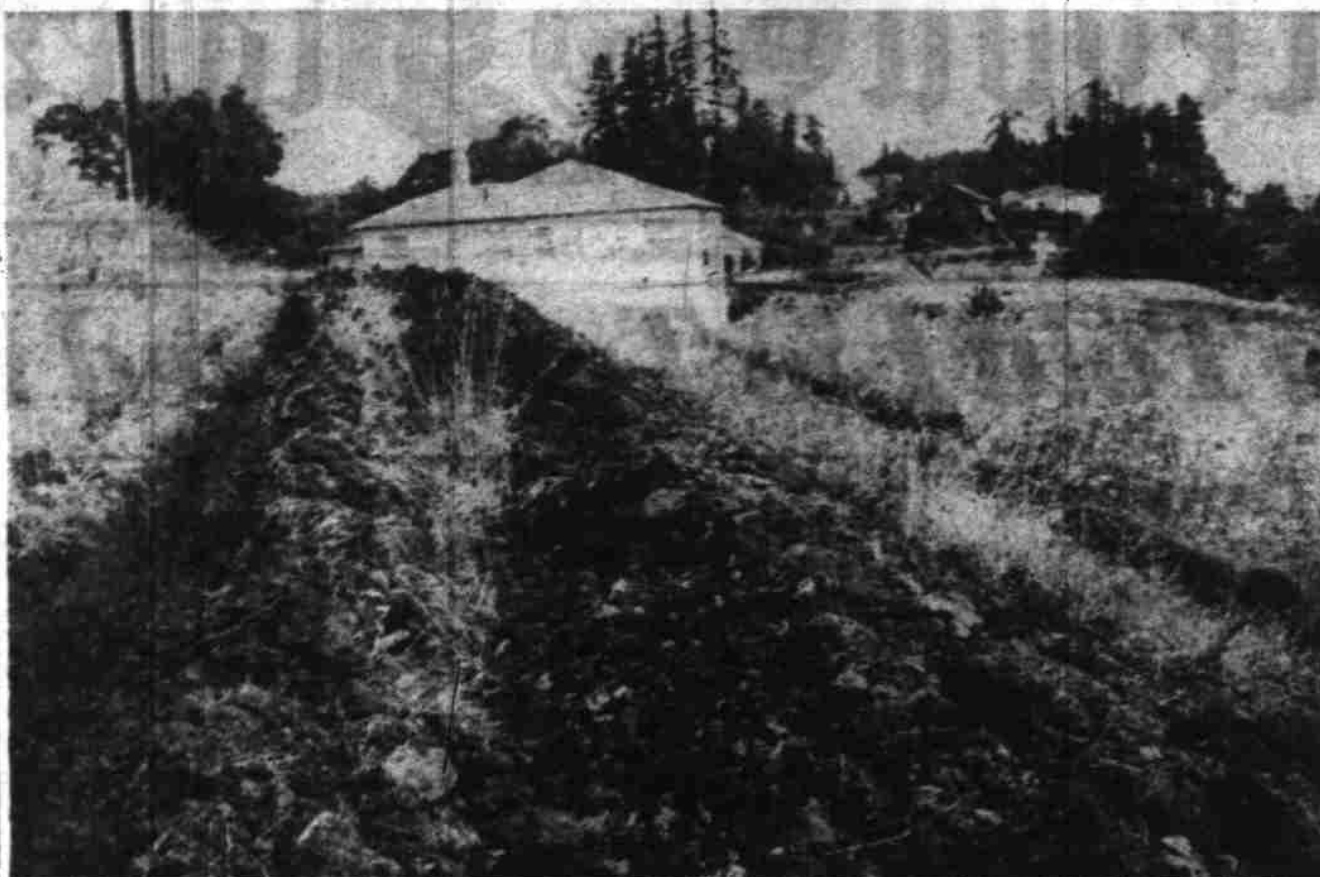
High and sometimes dry areas of Kingwood drive on the heights back of West Salem may not be quite so dry during drouth periods after an eight-inch water main is installed by the Salem water department. Current work on the main is shown above with some of the houses affected by the water shortage. The main will extend from the foot of Kingwood drive to Glen Creek road, and later an elevator tank will be installed to care for next summer's needs. (Statesman photo.)
