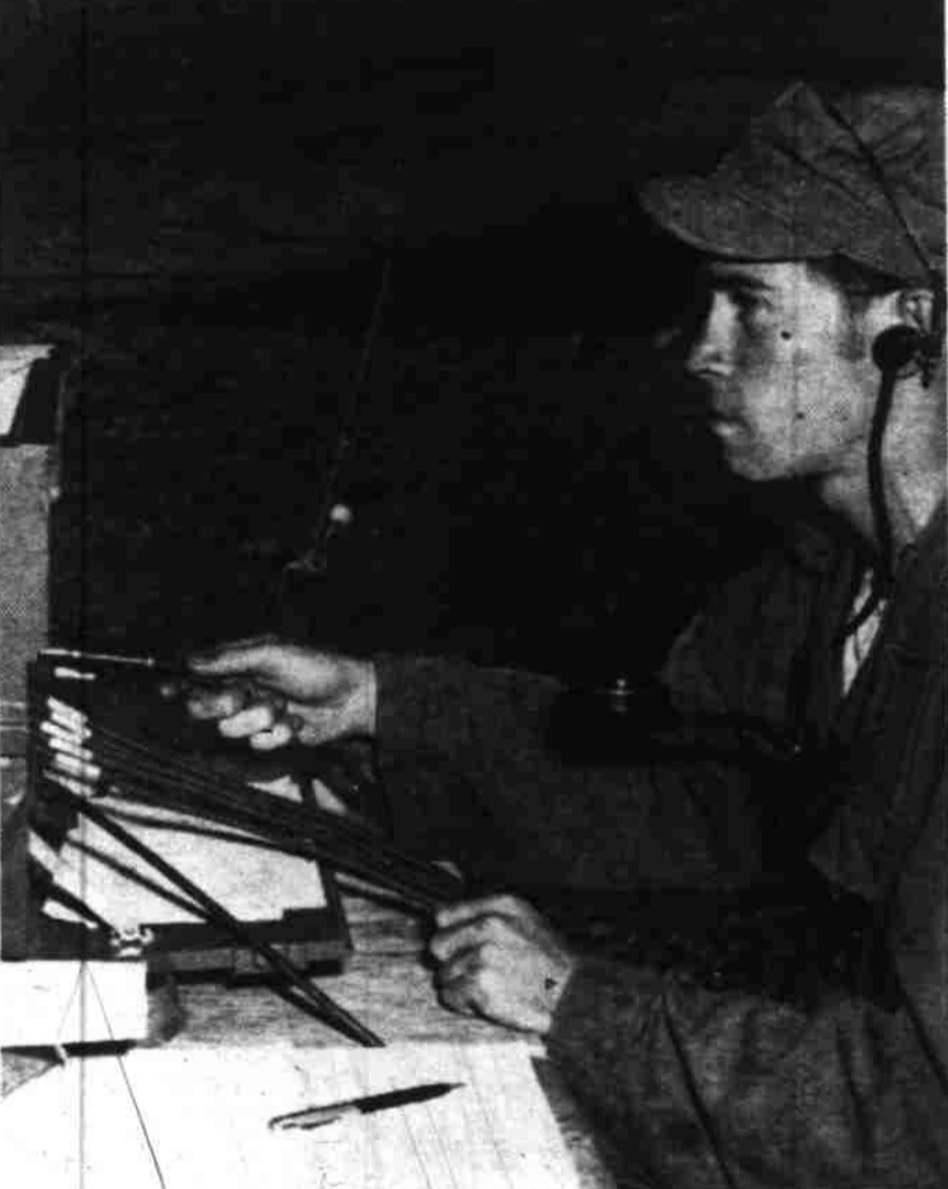
FT. LEWIS, Wash., June 20—Through the use of small field switchboards, such as shown here, battalion headquarters is able to be in constant communication with component units during national guard summer training here.
