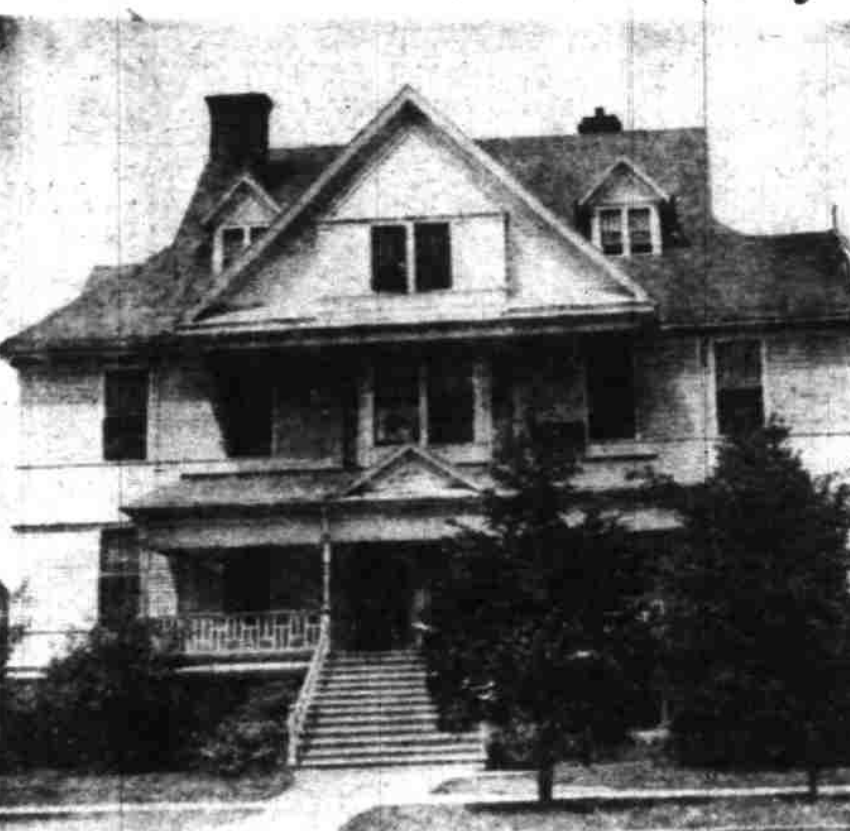
Next week will see Frederickson hall retired from use by Willamette university as a dormitory for students. The old three-story building was pressed into use by the university during the war housing shortage and this past year housed women students. It is located on the corner of South Winter and Ferry streets. (Statesman photo.)
