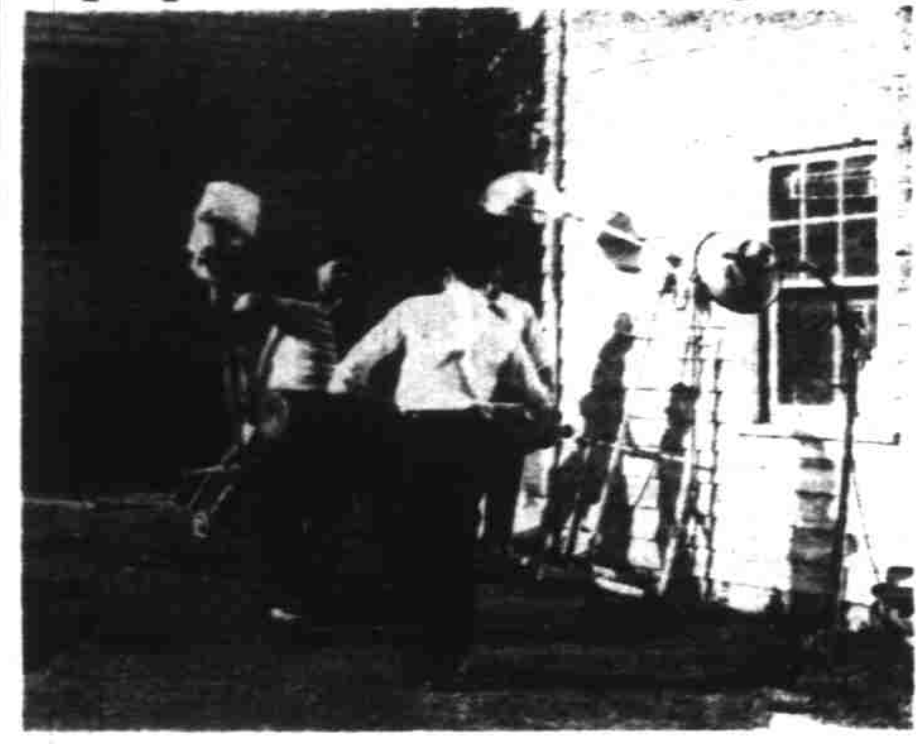
DALLAS, May 15.—Volunteers and firemen are shown removing valuable medical equipment from Dallas General hospital Sunday after a fire broke out in the building's attic. No one was injured and no equipment was lost. (Statesman photo). (Pictures also on page 1).
