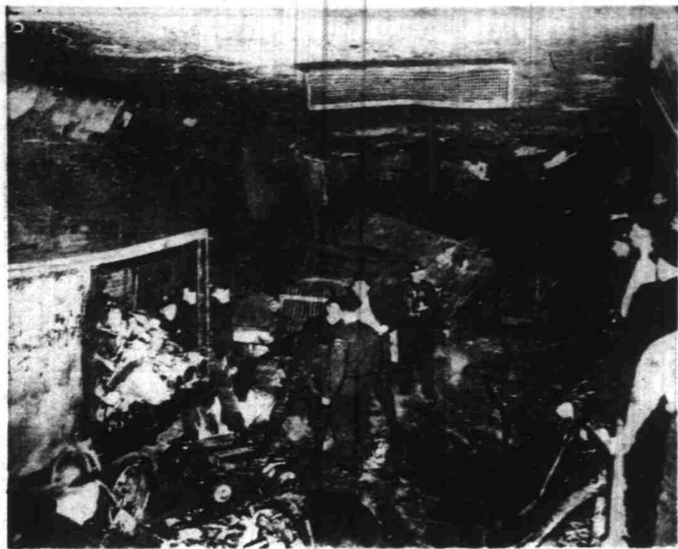
NEW YORK, May 13—Debris litters the Holland Tunnel's east bound tube today following explosion of drums of chemicals on a truck. Explosion was touched off when truck (center) caught fire near the New Jersey end of the tunnel. Flames spread to other trucks and the underpass highway was filled with carbon disulphide fumes. Firemen wearing gas masks brought the fire under control. (AP Wirephoto to the Statesman.)
