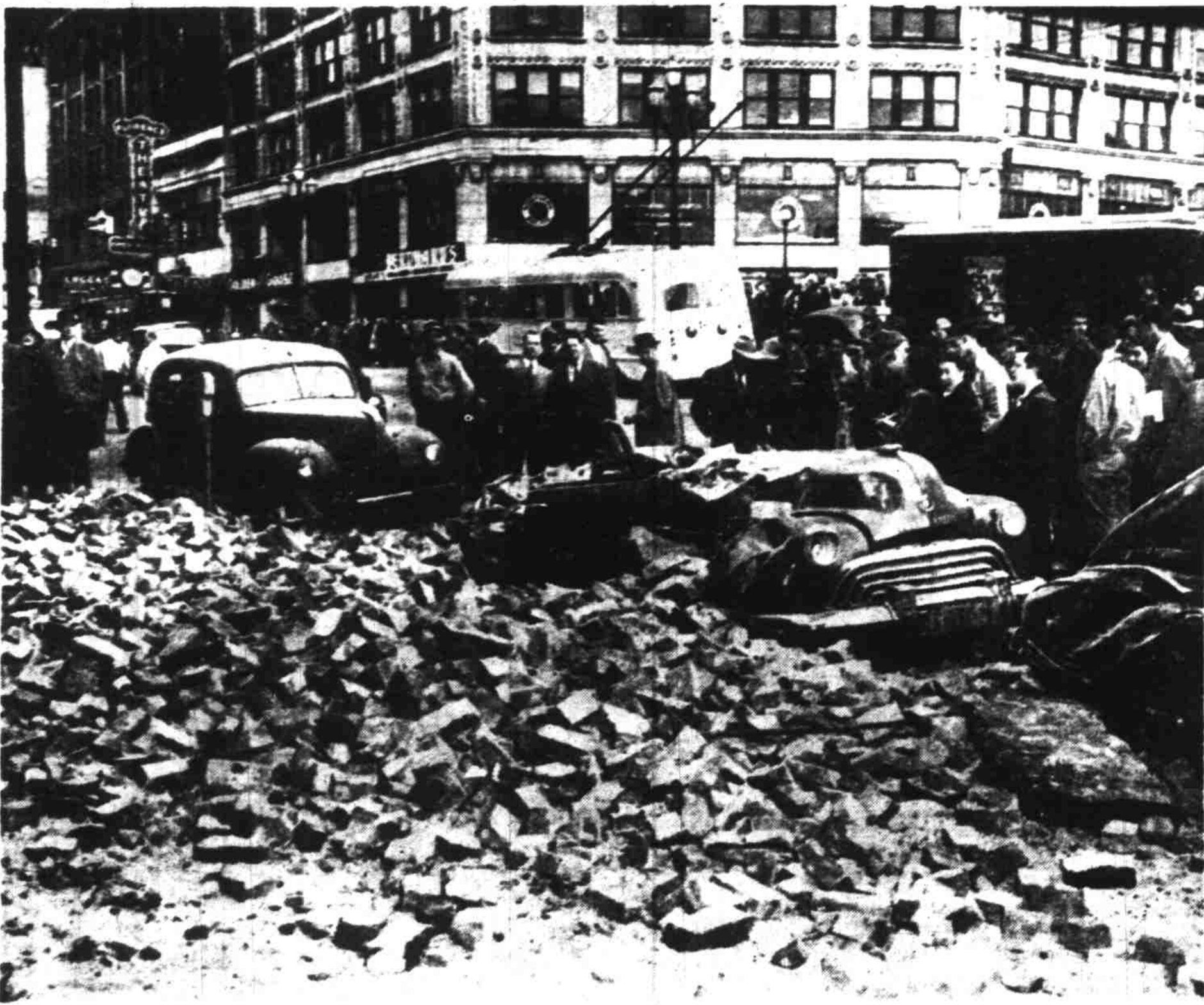
SEATTLE, April 13—This photo shows damage to automobiles from falling bricks in downtown Seattle during today's strong earthquake. (AP Wirephoto to The Statesman).
