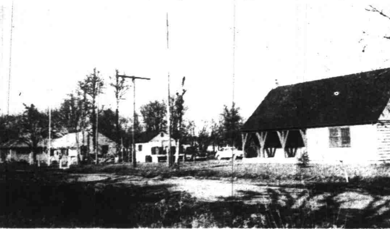
DALLAS—Headquarters of the Polk-Benton district, Oregon state board of forestry, in Dallas is shown above. Building in foreground is where crew of 10 to 15 men eat and sleep during the fire season. House-shaped building under construction will be administration building. At extreme left is warehouse which was recently completed. An equipment garage will be built next. (Statesman photo).
