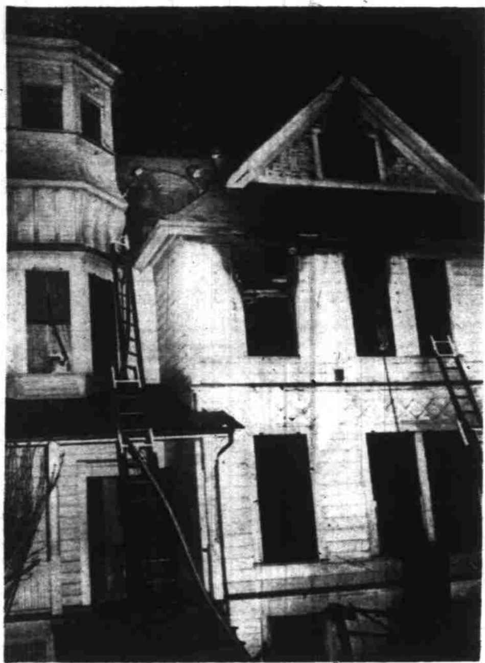
Three Salem firemen pass a hose into the turret windows of the old Chateau apartment house at 585 S. 12th st. while fighting a stubborn fire which gutted the two top floors Friday night. The firemen, left to right, are Walt Mills, Jack Johnson and Harvey Reinke. No one was injured in the fire which is believed to have started in a front apartment of two students on the second story at right. (Photo by Don Dill, Statesman staff photographer.)
