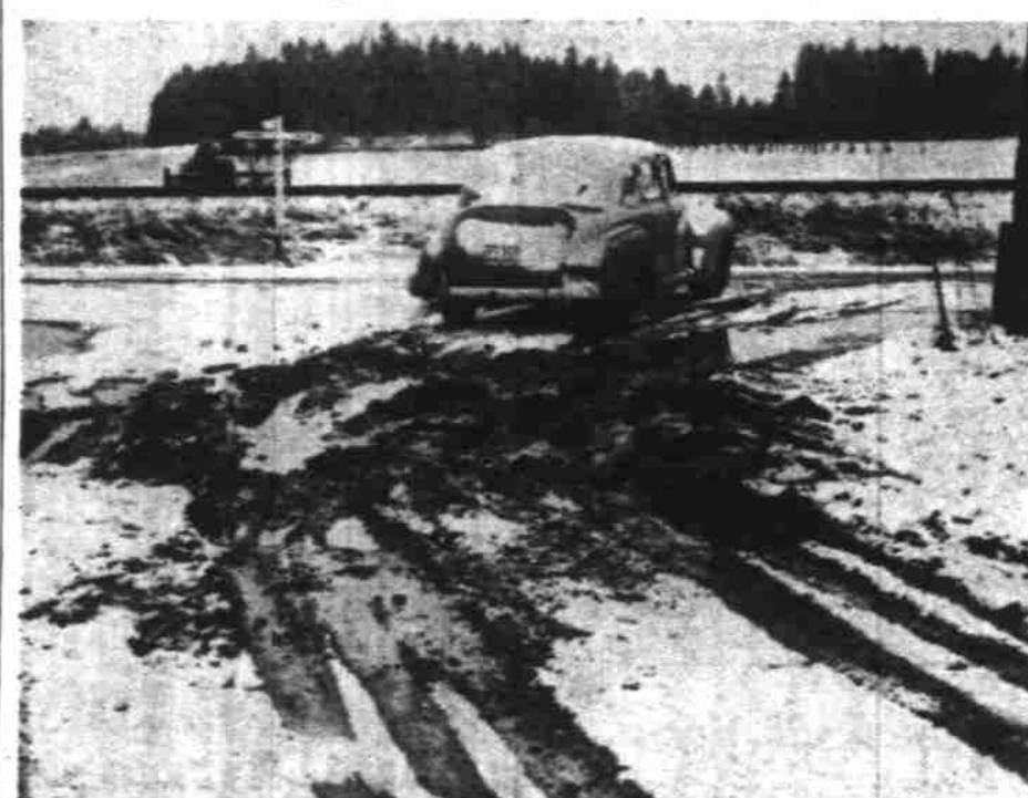
What once was a good, solid gravel road in Marion county is now only a quagmire with holes 20 inches deep. The intersection is of the Chemawa-Claxier roads. The same condition exists throughout the Willamette valley as a result of the long freeze. (Statesman photo). (Additional photos on page 5).
