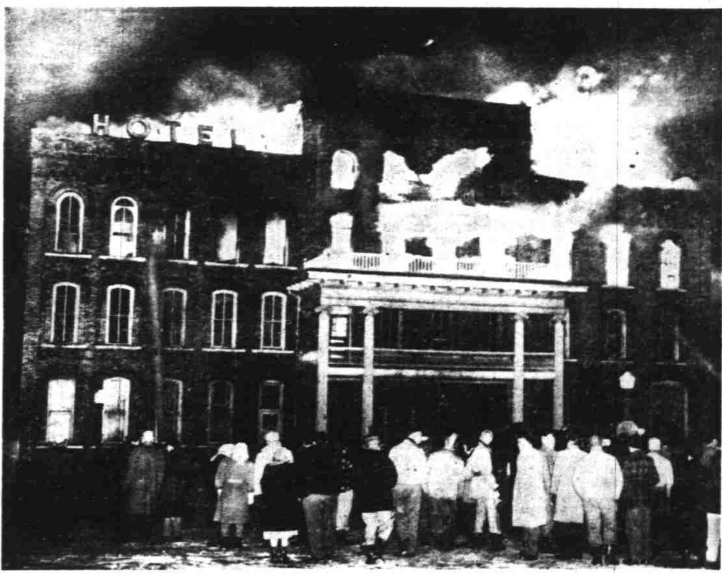
RIPON, Wis., Feb. 1—Flames shoot from the roof and windows of the historic Grand View Hotel which was destroyed early today. More than 40 guests escaped but authorities listed six persons as missing and presumed dead. The cause of the fire was undetermined. (AP Wirephoto to The Statesman). (Story on page 2).
