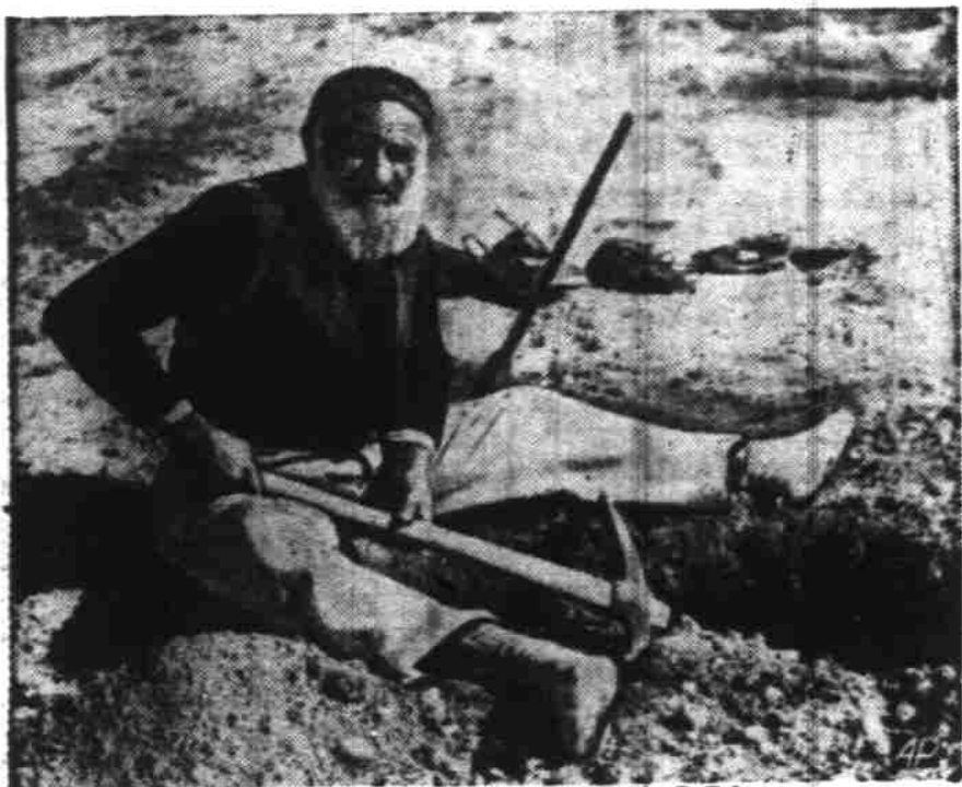
ON THE "ROAD OF COURAGE" —An elderly Jew takes a rest from his digging while at work on the new Jerusalem-Tel Aviv highway called the "Road of Courage."
