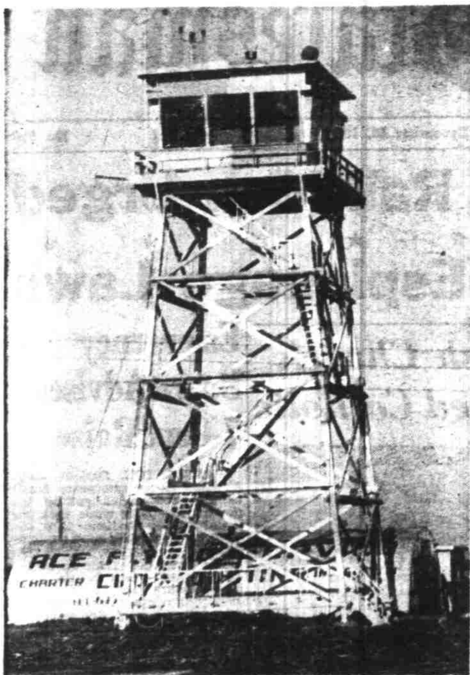
Salem's aerial future will be shaped with the opening of the aircraft control tower pictured above. Closed since the war except during last spring's flood emergency the tower is now being renovated for operation by the civil aeronautics authority. The quonset hut at its base is being remodeled for heavy equipment and offices. Six men will work the tower on a 24 hour basis. (Photo by Don Dill, Statesman staff photographer.)
