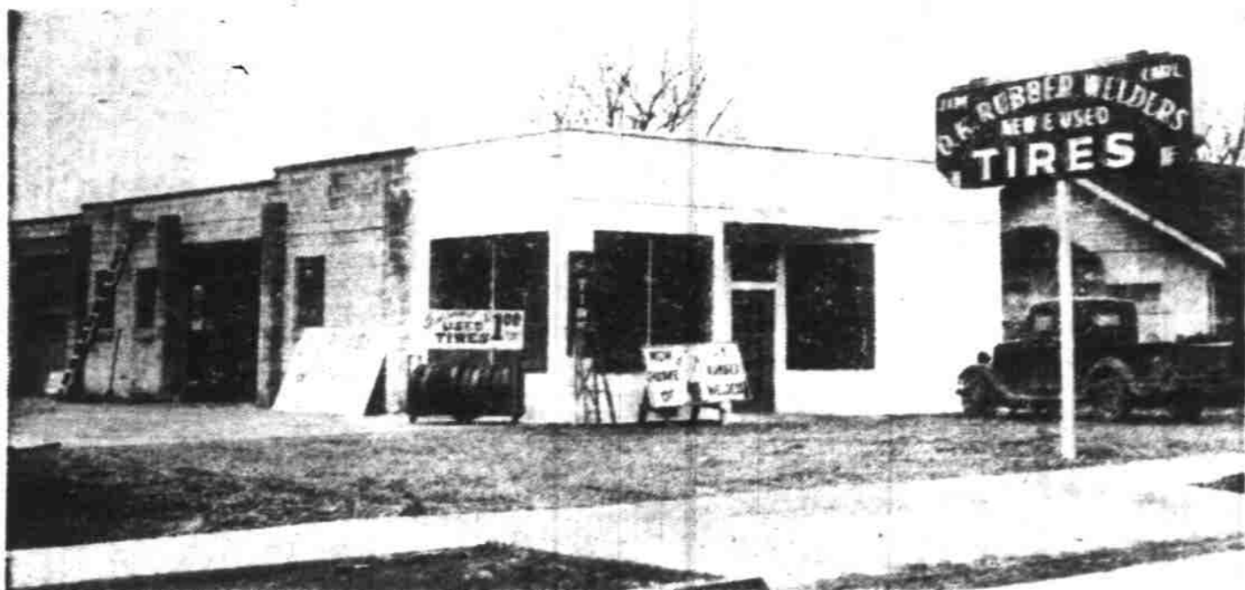
This is the new home of O. K. Rubber Welders at 1820 S. 12th st. The business is owned and operated by James Sidwell, veteran rubber vulcanizer who operated at 202 S. High st. for 12 years before moving into the new building. Sidwell said the factory combines the latest vulcanizing and rubber welding equipment. (Photo by Don Dill, Statesman staff photographer.)
