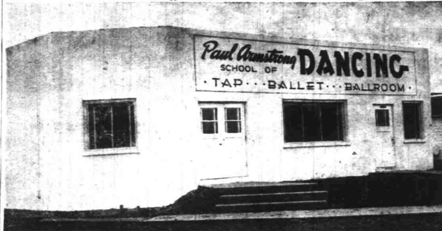
Shown above is the recently completed home of the Paul Armstrong School of Dancing at 1990 Mission st. The new dance studio houses an office, dressing rooms for boys and girls, an auditorium and stage for programs and a glass-windowed reception room for parents who wish to watch their children learn dancing. The school formerly was located in downtown Salem. (Photo by Don Dill, Statesman staff photographer).
