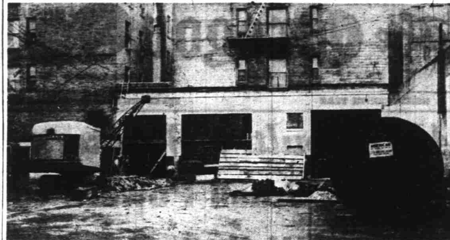
Remodeling of the Senator hotel has moved to the rear area formerly occupied by the Greyhound bus lines. Shown above from the alley is the space where buses loaded and unloaded, the canopy torn down and workers busy ripping up the concrete. At right is an oil tank which will be buried. Dining and lounge rooms will go into the vacated part of the hotel building. (Photo by Don Dill, Statesman staff photographer.)
