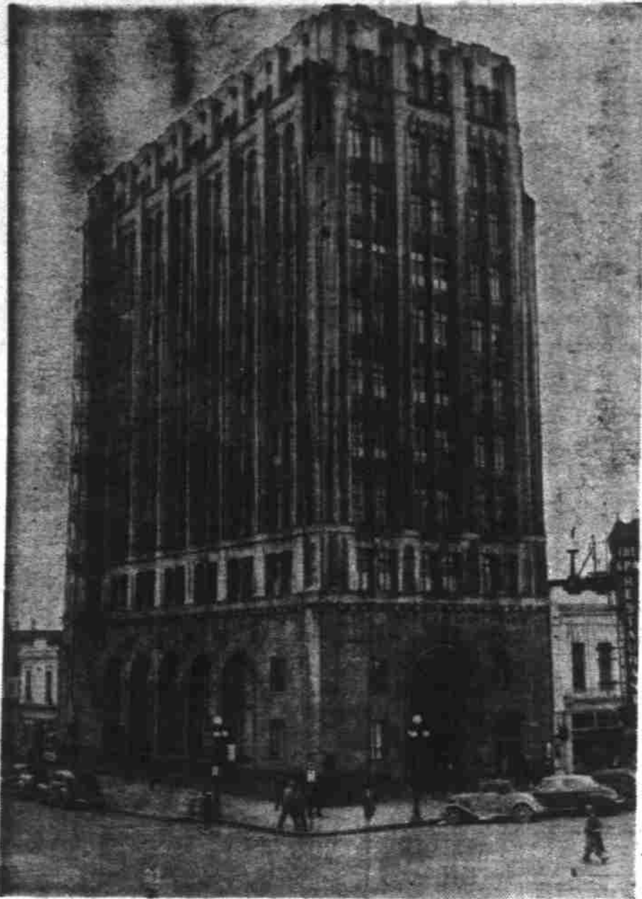
The T. A. Livesley building at State and Liberty streets, Salem, the entire ground floor of which was leased for 15 years Thursday by Stevens and Son, Jewelers.
