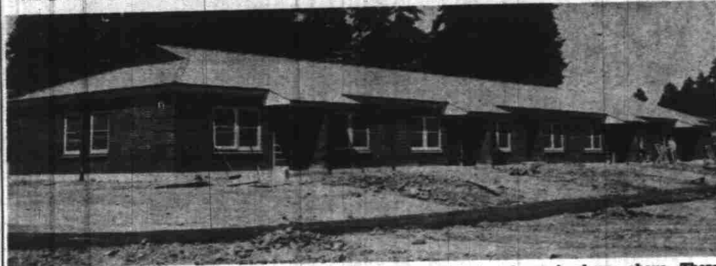
One of the two married employes' cottages just finished at Fairview home is shown above. There are eight two-room apartments in each of the two married couple cottages and accommodations for 16 in a new single nurses' cottage. A total of 48 employes will be housed in the new buildings.
