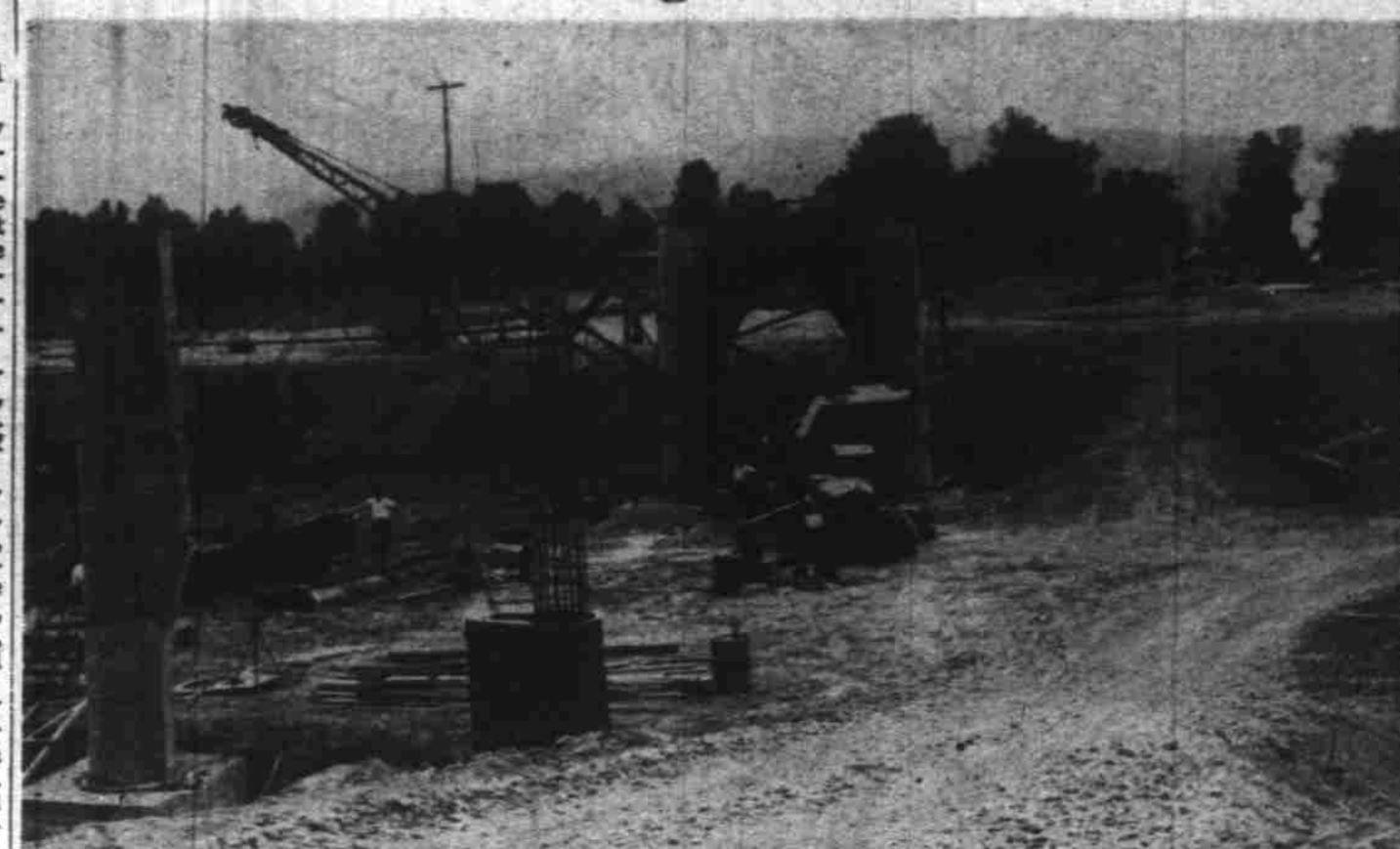
INDEPENDENCE, Aug. 9 — Work is progressing on the concrete footings for the new Marion-Polk county bridge at Independence as shown in the above photo, taken from the Independence side of the Willamette river. Steel forms are used to mold the graceful arches of the piers, and the crane is necessary to move the heavy forms into place. Construction is by the Macco Co., of California. (Photo by Don Dill, Statesman staff photographer.)
