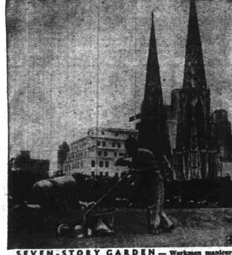
SEVEN-STORY GARDEN — Workmen manure a lawn and garden on seventh floor of La Maison Francaise, one of the fifteen buildings of New York's Rockefeller Center. The spires of St. Patrick's Cathedral are in background.
