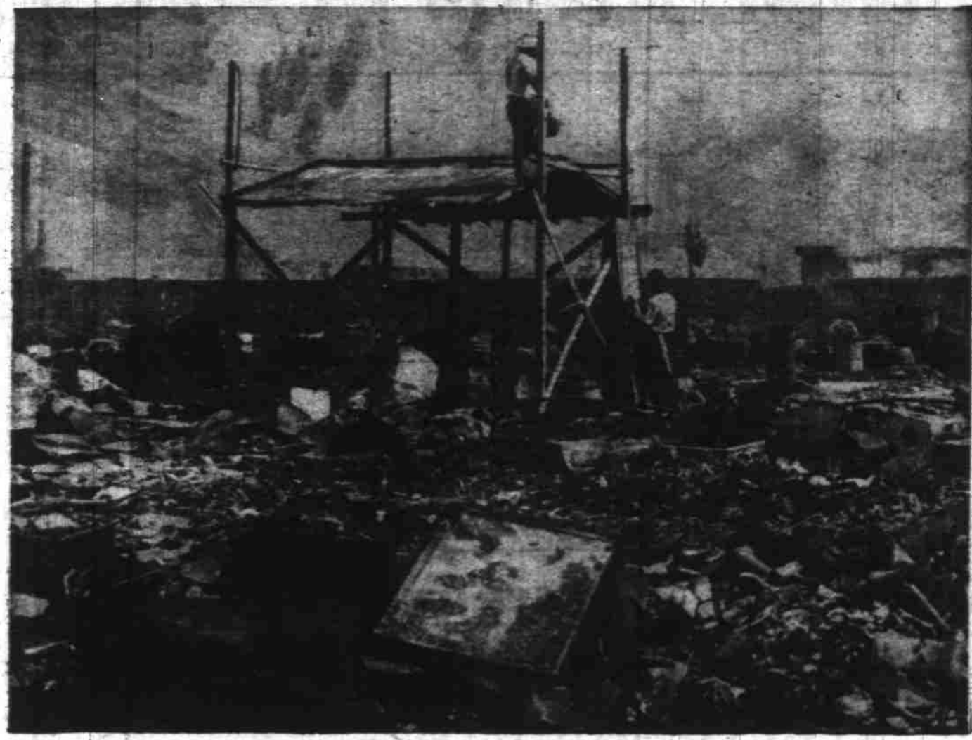
FUKUI, Japan, July 2—Residents of Fukui, Japan, build a temporary structure amidst wreckage within hours after a disastrous earthquake and fire swept the industrial town. Photo made by Charles Gerry, Associated Press Staff Photographer, who flew to the scene from Tokyo. (AP Wirephoto to the Statesman.)
