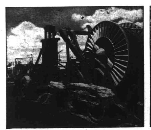
2. We plant "co-ax" with giant plows like this. Every eight miles a "booster station" keeps calls going through clearly. For - incredible as it seems - high frequency waves fade so rapidly in the cable that all the sun's energy, if it could be funneled into the pipes, would not earry half-way across the country.
