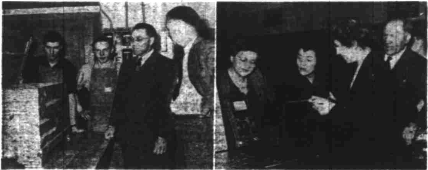
Cabinet and furniture work are favorites of students in the woodworking shops of Salem High school. Photo at left shows a fine cedar chest under construction, exhibited to Lester A. Wilcox, assistant state superintendent of public instruction, at right, during the high school vocational shops' open house Monday afternoon. Others are, left to right, Dean Jones, 1130 Spruce st.; James Vibert, route 7; and M. H. Davis, shop head. In photo at right, high school instructors are shown taking a personality test on a special meter rigged up by the radio and electronics shop students. Pictured are, left to right, Mrs. Gertrude Shiller, algebra instructor; Margaret Burroughs and Mrs. Grace Hockett, both English instructors; and C. R. Lindstrom, vocational director. (Photos by Don Dill, Statesman staff photographer.)
