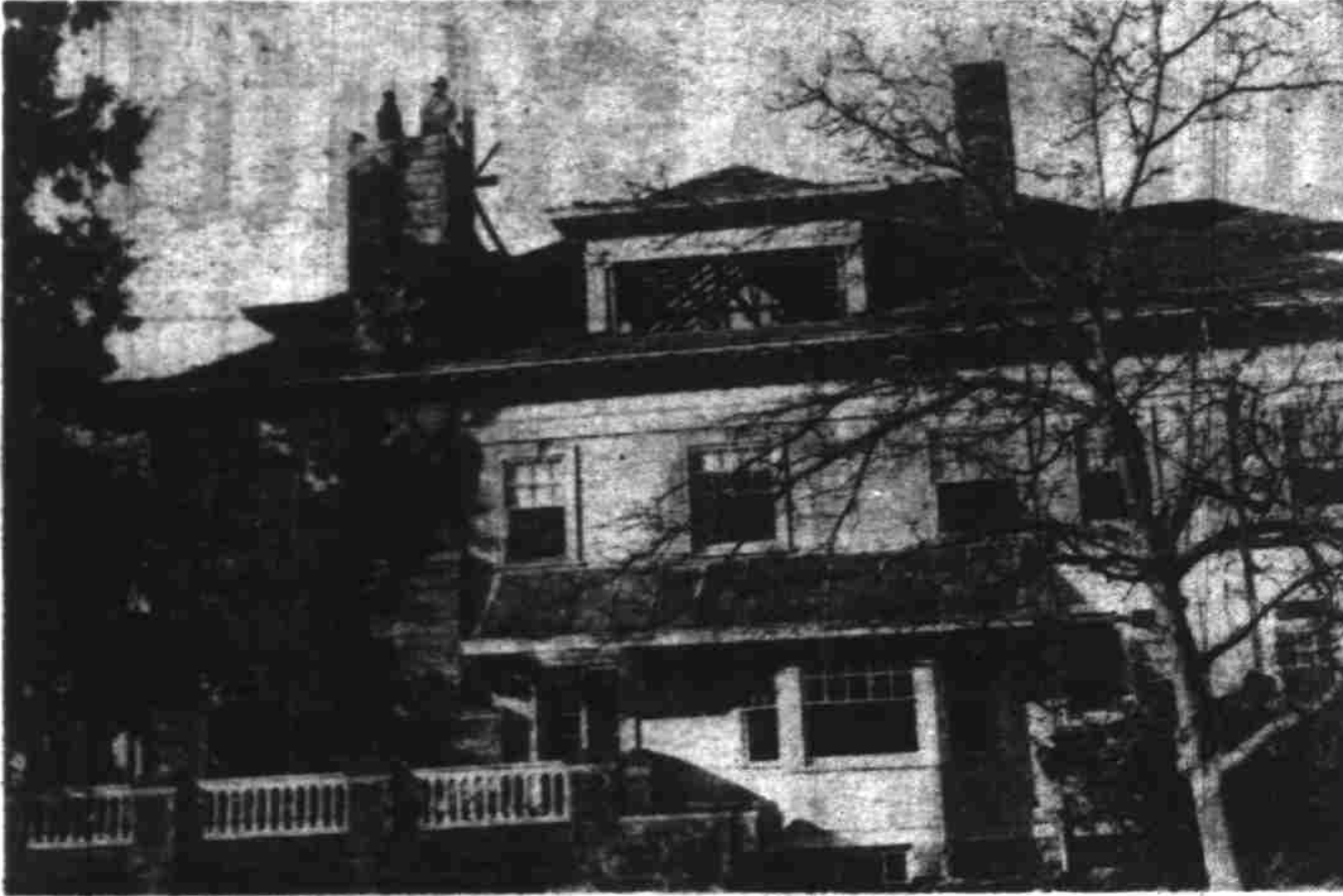
A new Oregon state office building will rise on the site of the old B. C. Miles home, 993 Court st., shown above being dismantled by workmen, and the Charles K. Spaulding home beside it. For many years the Miles and Spaulding homes were regarded as among the more palatial homes in Salem. Furnishings such as fine wool paneling and leaded windows as well as the fixtures are being sold on the spot by wreckers. The pastoral scene on the tile fireplace (lower photo) was painted by Lyra Miles, daughter of B. C. Miles. Chris Madsen, who was awarded the job of wrecking the Miles home for $911.14 and the Spaulding home for $711.12, is shown above preparing to dismantle the fireplace. (Photos by Don Dill, Statesman staff photographer.)
