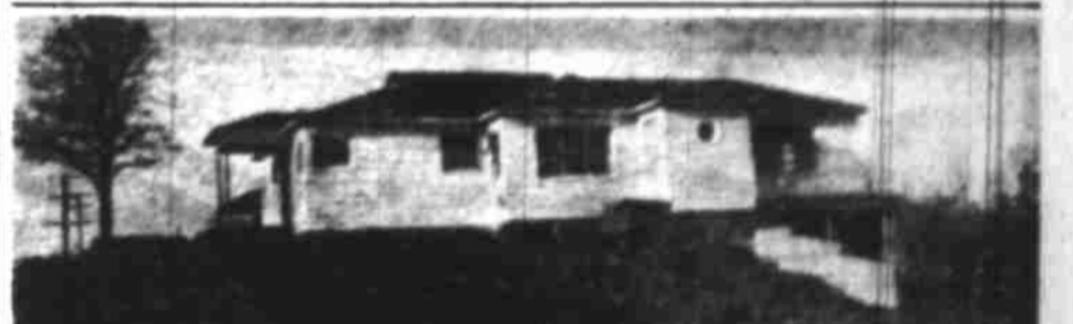
Nearly Ready for occupancy; View, large lot, dining R., basement with garage, bk. book, 3 B. E. Max. F. R. A. loan avail. 674 E. Ewald near 99 or Ph. 8861.
