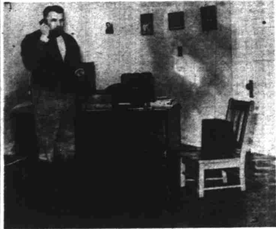
It was Waters field literally yesterday as flood waters covered the entire playing field with depths of two and three feet of the raging aqua. Even the office premises didn't escape as the above picture indicates. It shows Senators Business Manager George Emigh, almost knee deep in water, calling the weather bureau for a report on what he can expect next. (Don Dill Photo, The Statesman).
