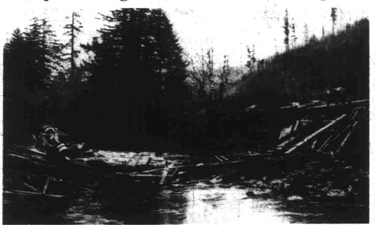
This upended logging truck and collapsed bridge were the result of a Tuesday accident at Lumber bridge over the Little North Fork of the Santiam near Mehama. Driver Arthur Anderson of Lyons escaped with minor injury when the bridge collapsed as he was crossing it. A Bailey-type army bridge of steel will temporarily replace the Lumber bridge, county officials said Wednesday. The above photo was taken by Raymond Vitato, 225 S. Lancaster dr., Salem, who was a passerby at the time of the accident.
