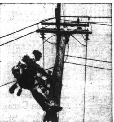
Power-line carrier is another new device which makes telephone communications possible in remote, sparsely settled districts. Your voice "hitch-hikes" along existing power lines on radio waves that are tuned to follow the wires. Several power-line systems are now used on the Pacific Coast . . . and they're as safe and effective to use as any.
