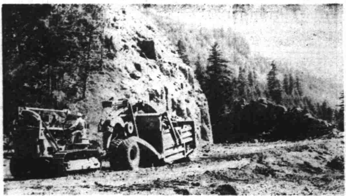
With the first relocated section of the North Santiam highway due to open to the public this month, final road work over the $475,000, 4 1/2-mile stretch east of Gates is being rushed by the Kackenberg Construction Co., of Portland. In photo above Al Benson is operating a huge 25-yard LeTourneau scraper at a point 2 1/2 miles east of Gates on a slightly higher level than the present road. A railroad crossing will be eliminated at this location. Edward Pinkston has charge of the road construction between Gates and Niagara, where rolling and filling are now in progress. (Statesman photo by Don Dill, staff photographer).
