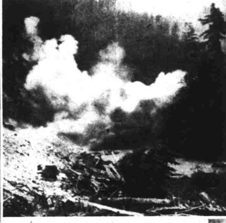
This explosion (top left photo) Friday evening blasted nearly 40,000 tons of rock from a bluff (middle left photo) over the North Santiam river two miles east of Niagara and 3 1/2 miles west of the site for the Detroit dam. The Kuckenberg Construction Co. of Portland, which is relocating the North Santiam highway from Gates to Detroit, used 5,500 pounds of dynamite to make way for the new highway which is to be at river level here, then rise over the next few miles to the top of the 350-foot-high proposed dam. Middle right photo looks down from the 175-foot bluff on heavy construction equipment as earth was packed on railroad tracks as protection a few minutes before the blast. River shows in background. Lower photo shows the crushed rock and separated boulders (later dynamite) which spilled over into river, as clearance work began to reopen railroad this week. (Statesman photos by Don Dill, staff photographer.)
