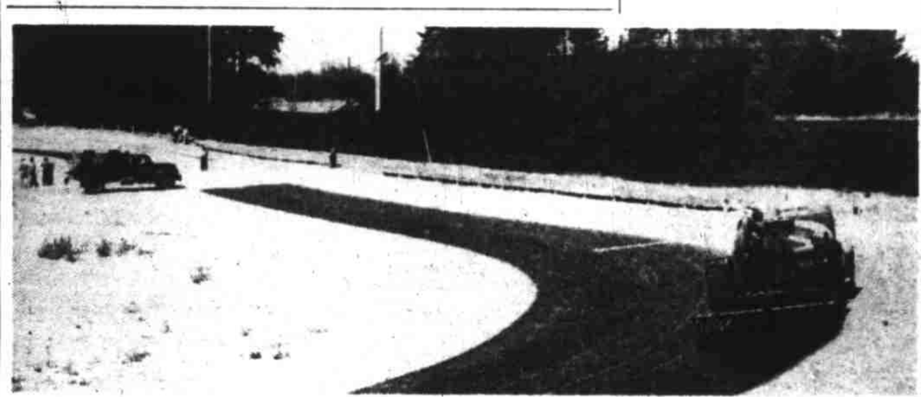
The Hollywood Bowl premises north of town have been undergoing a first-rate manuevering lately, making ready for the midget auto racing inaugural tomorrow night. A $10,000 track paving job and the building of the 3000-plus capacity grand stand, pictured above, kept the workmen busy. Racing men opine the quarter-mile oval will be the fastest on the Pacific coast. (Don Dill photo, The Statesman.)
