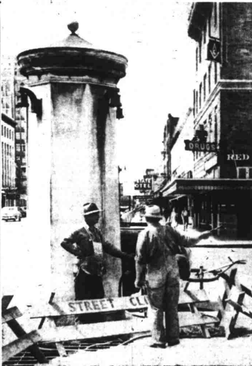
Another downtown Salem landmark soon to be gone is the ventilation tower of the underground rest rooms on the northeast corner of State and High streets, as work of widening High street progresses. Shown at the left with an air hammer is Leslie Walker, Salem route 3, as William Neal, 995 S. 14th st., points with his hammer while the two discuss the work. (Photo by Don Dill, Statesman staff photographer.)
