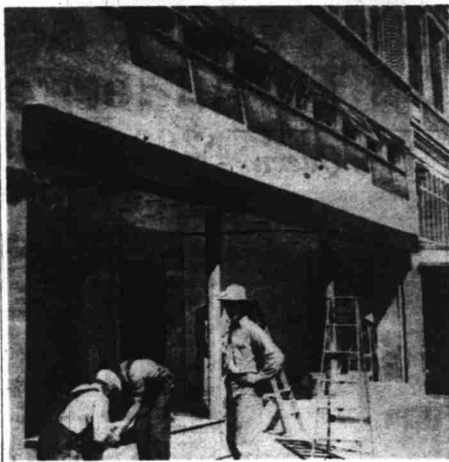
Finishing touches are applied by workmen to display windows in the modernistic front of the Schlesinger and Co. women's apparel store, 469 Court st. The remodelled store is expected to reopen next week. (Statesman photo by Don Dill, staff photographer.)
